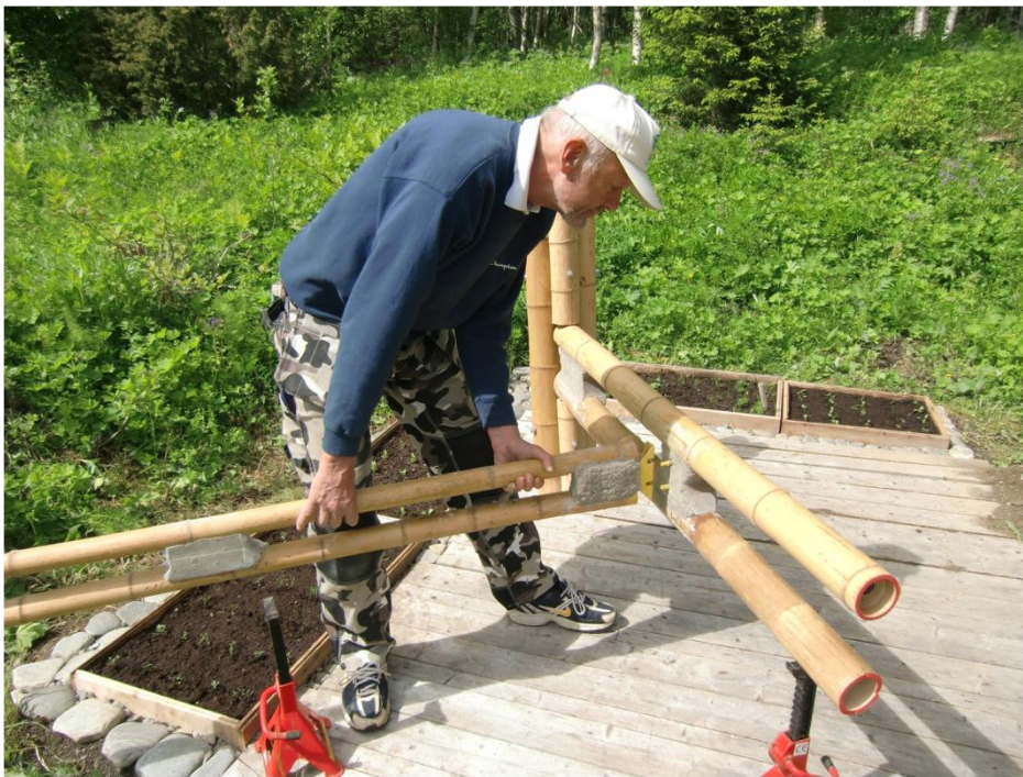
Mounting of a prefabricated floor joist
