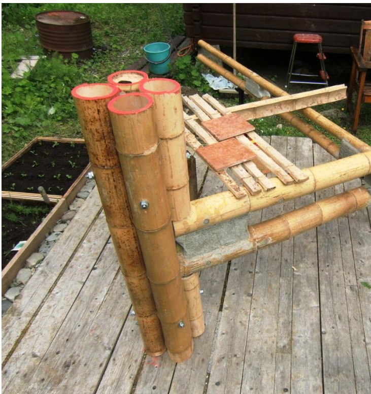
Buildup of a multistory structure
