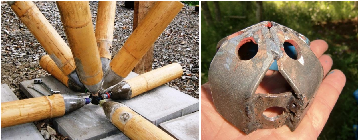
The “Pet Crown” space frame connector for eight elements converging into one moment free point. Architect: Ingemar Saevfors, 2012
