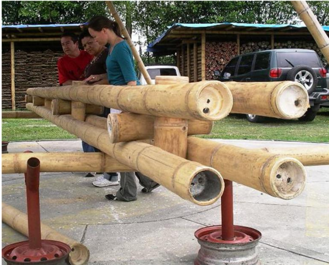
Assembly of a Spaced Column resistant to buckling, with Joerg Stamm at Eco-Bamboo, Colombia, 2009.
